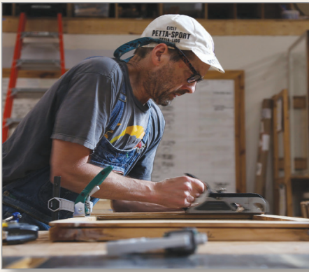
Mozer Works Inc. founder and principal Neil Mozer restores a wood window sash. Photo by Jeff MacMillan
