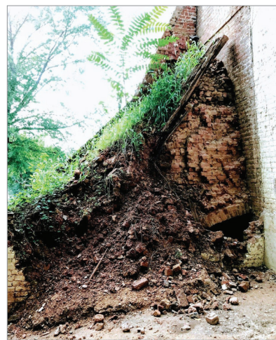
Buttress, view of east elevation after east wall collapse, September 2017. Daniel Tana.
