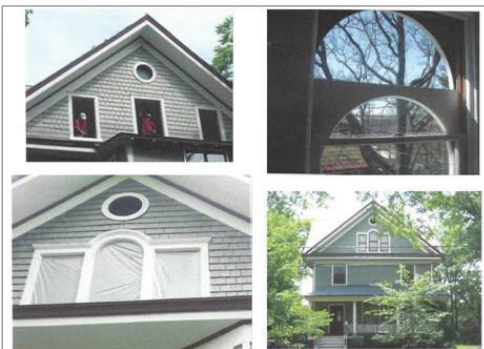
7121 Willow Avenue • Takoma Park, MD – $18,709.90 Window Restoration: Sashes, Sash Cords, Weather-Stripping, Hardware
