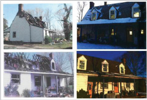
Chiswell's Inheritance 18200 Beallsville Road • Poolesville MD – $43,424.00 In-Kind Replacement of Roof Following Fire
